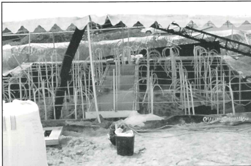
The test tank designed by NMTech researchers at the Oregon LEAP site.
